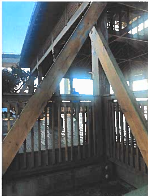
Photo 2 – Rear left side temporary bracing
