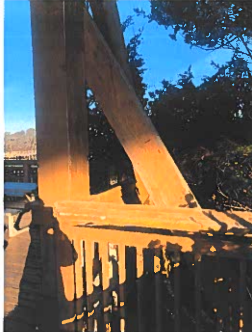
Photo 1 – Rear right side temporary bracing
