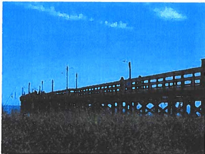
Pier and the Atlantic Ocean located at the Subject's "rear"
