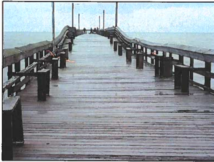
Figure 17. Example of timber decking
