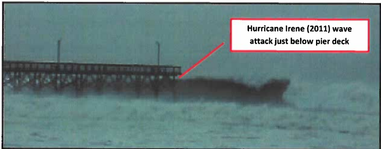
Figure 18: Wave heights just below pier deck during Hurricane Irene (2011).
