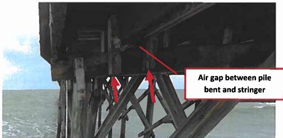
Figure 16. Example of timber bracing (red arrows) used to connect stringers to pile bents. Pile attached to pile bent by metal strap. Note that one of the stringers is not sitting on the pile bent in this photo.
