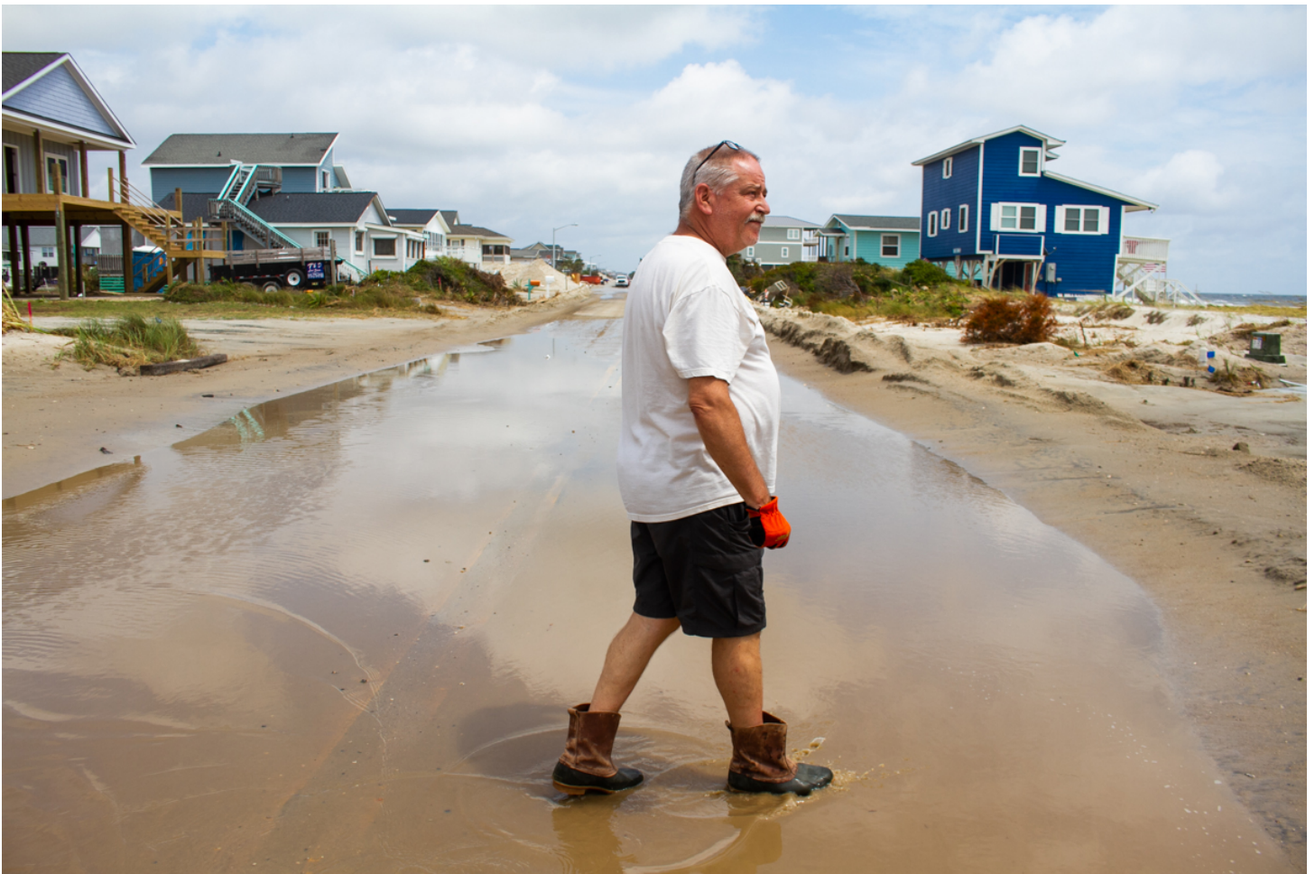
John Clift walks across flooded Beach Drive on Oak Island after Hurricane Isaias. “They should have never built on these lots,” he said of the oceanfront homes that removed dunes in front of his house. (Port City Daily photo/Johanna F. Still)
