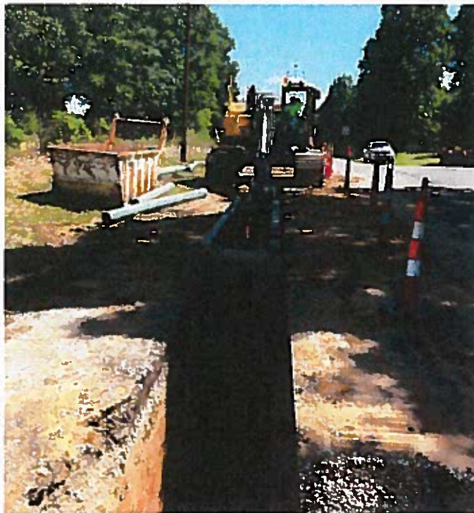
White House Sewer Project
