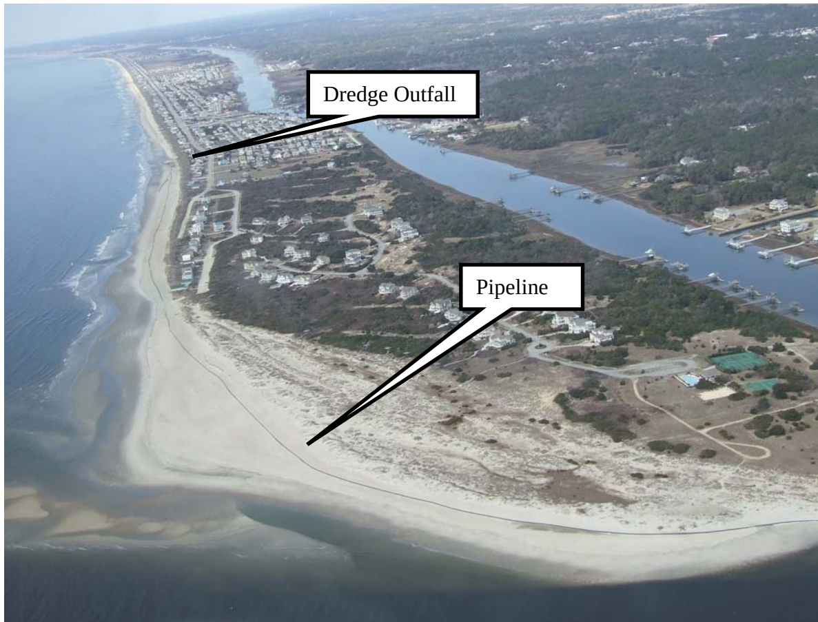
Figure 2-4. Aerial Photograph of Ongoing 2014 Nourishment (source: NCDQM)
